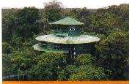
At the Aniau Towers, the largest of the Amazon tree lodges, guests can view flora and fauna from a unique perspective in the jungle canopy.
